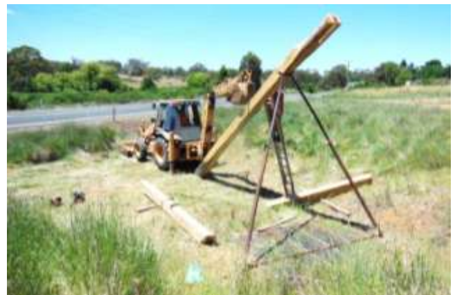
Installation of the replica headframe, Nov 2014
