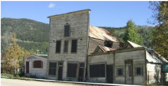
Dawson City- These buildings, long abandoned, are tilting because of the permafrost melting beneath their foundations
