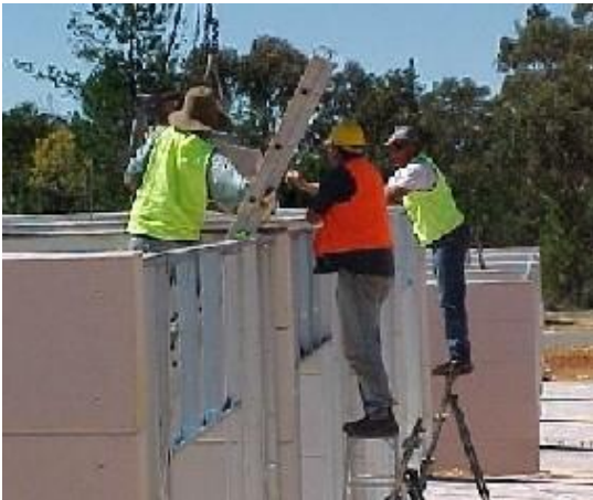
Motel Roofing Crew at work
