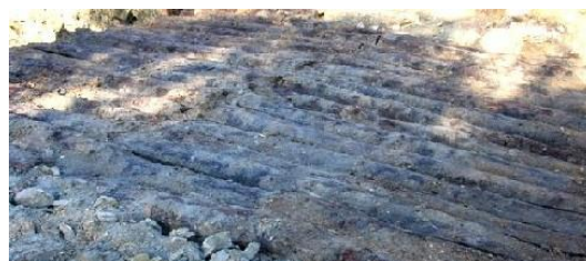
Exposed timbers of Germantown Lane Bridge
