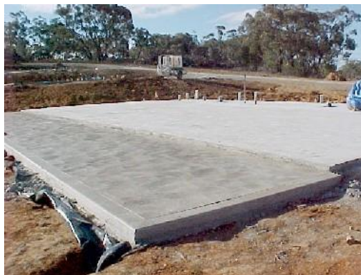
Concrete slabs for Hill End Motel
